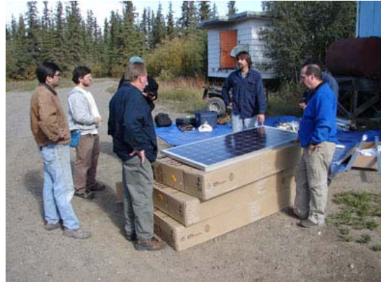
Solar panel installation in Fort Yukon
